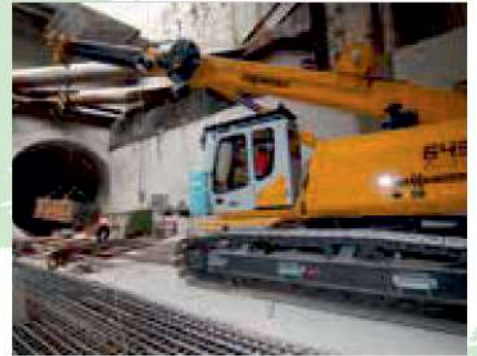
Tunnel construction Tunnelbau
