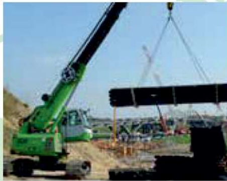
Civil engineering Tiefbau
